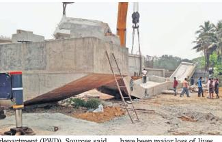
department (PWD). Sources said that fault in construction led to the collapse of the bridge. They informed that within 14 hours of the girder being placed on the pillars, the bridge collapsed. The sources also said that usually 50-60 labourers are present at the construction site. Luckily that was not the case Wednesday otherwise there would
