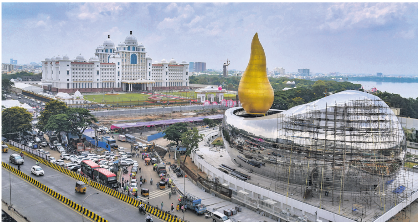
The new Telangana Secretariat building, on the day of its scheduled inauguration in Hyderabad, Sunday
