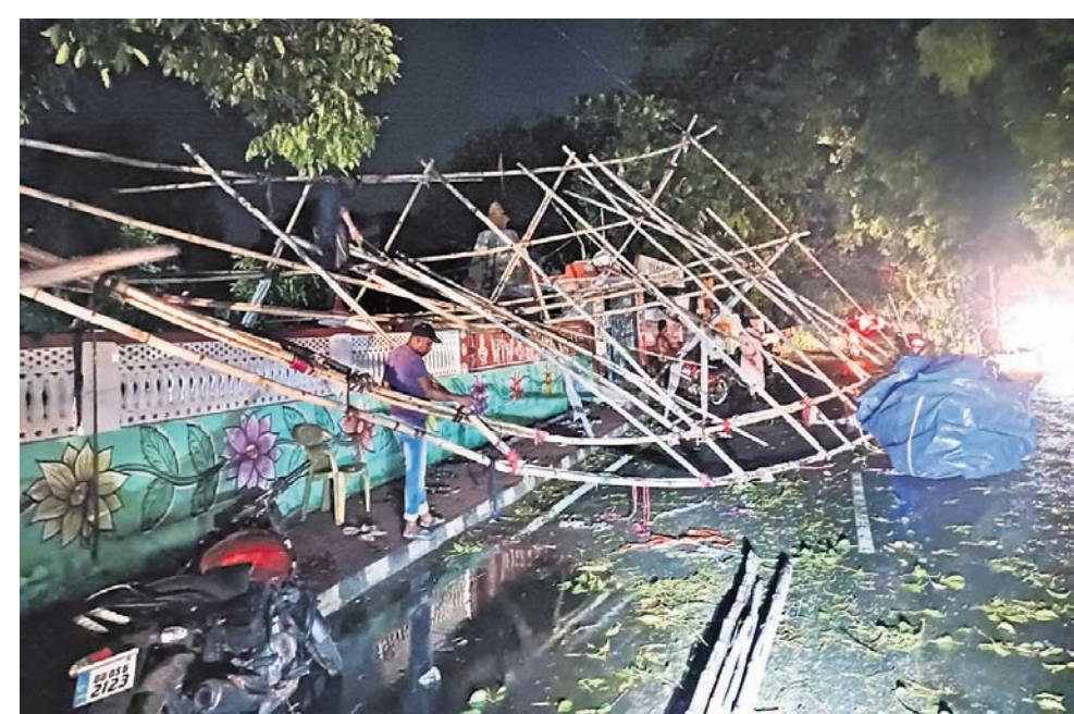
NATURE'S FURY: A bamboo structure erected at Chahata Ram Mandir came crashing down following rain and gusty winds in Cuttack, Friday
