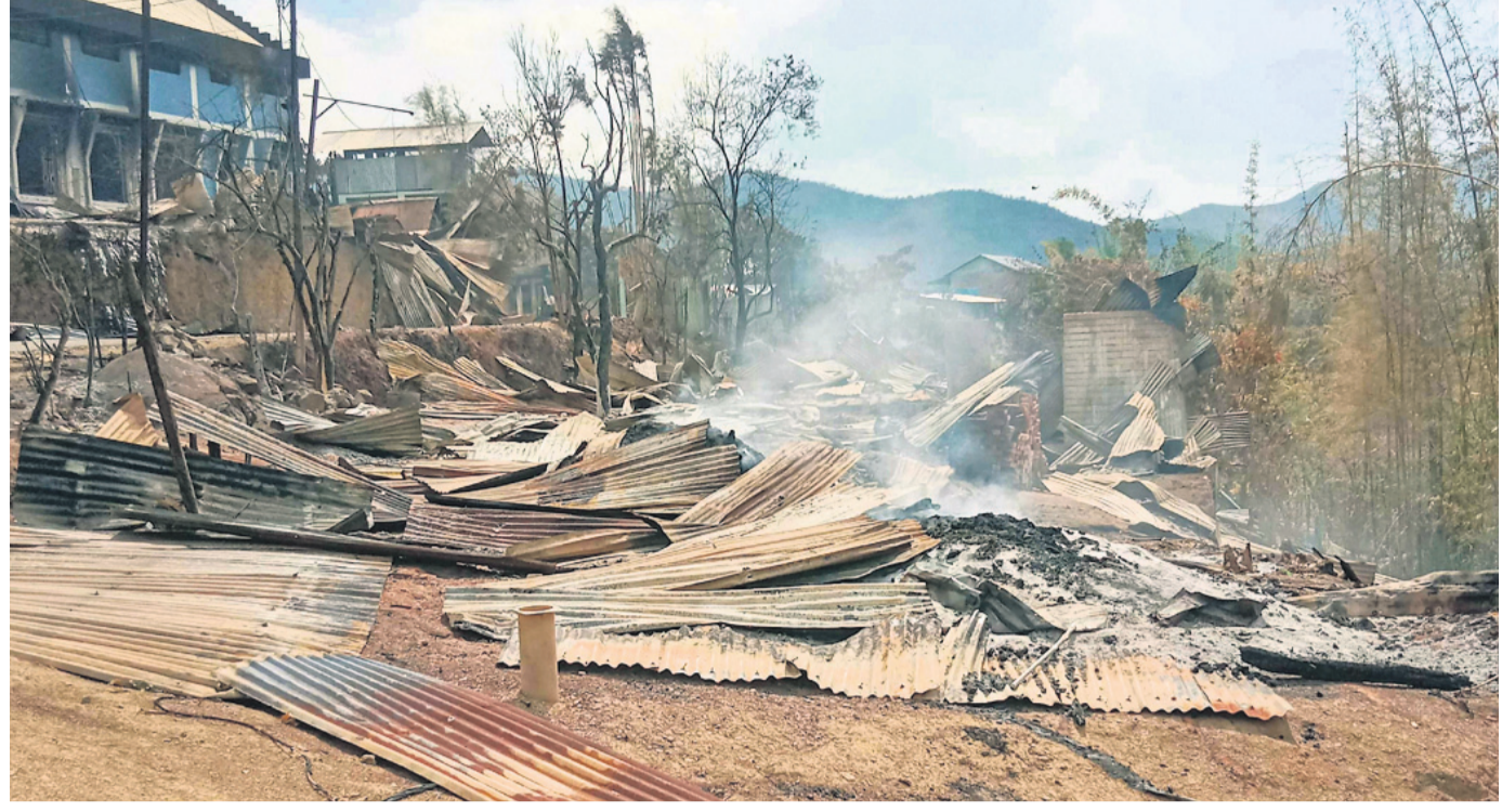
SMOKE & SCARS: A view of damaged house at violence-hit area of Sugnu, in Kakching district of Manipur, Wednesday
