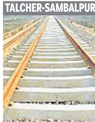
Sambalpur Division Tuesday. Chowdhary inspected safety-related aspects like overhead equipment, bridges, signal & telecom-
