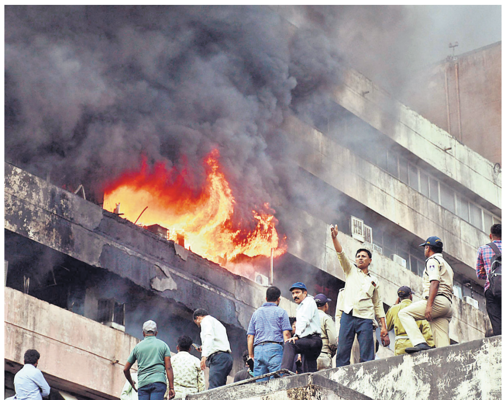
RAGING INFERNNO: Firemen douse a blaze that broke out on the third floor of Satpura Bhawan, a building housing offices of various departments of the Madhya Pradesh government, in Bhopal PTI PHOTO
