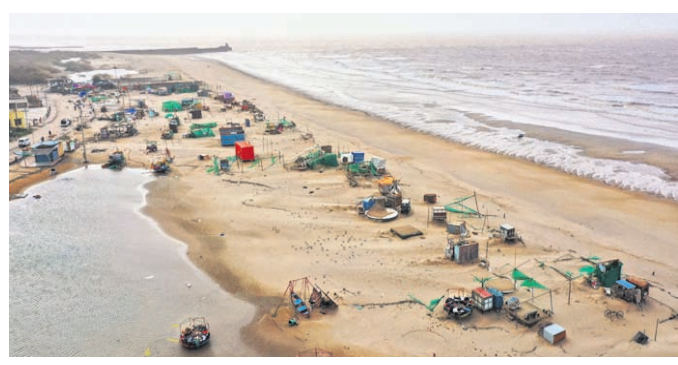
Damaged temporary structures at a beach in Mandvi
