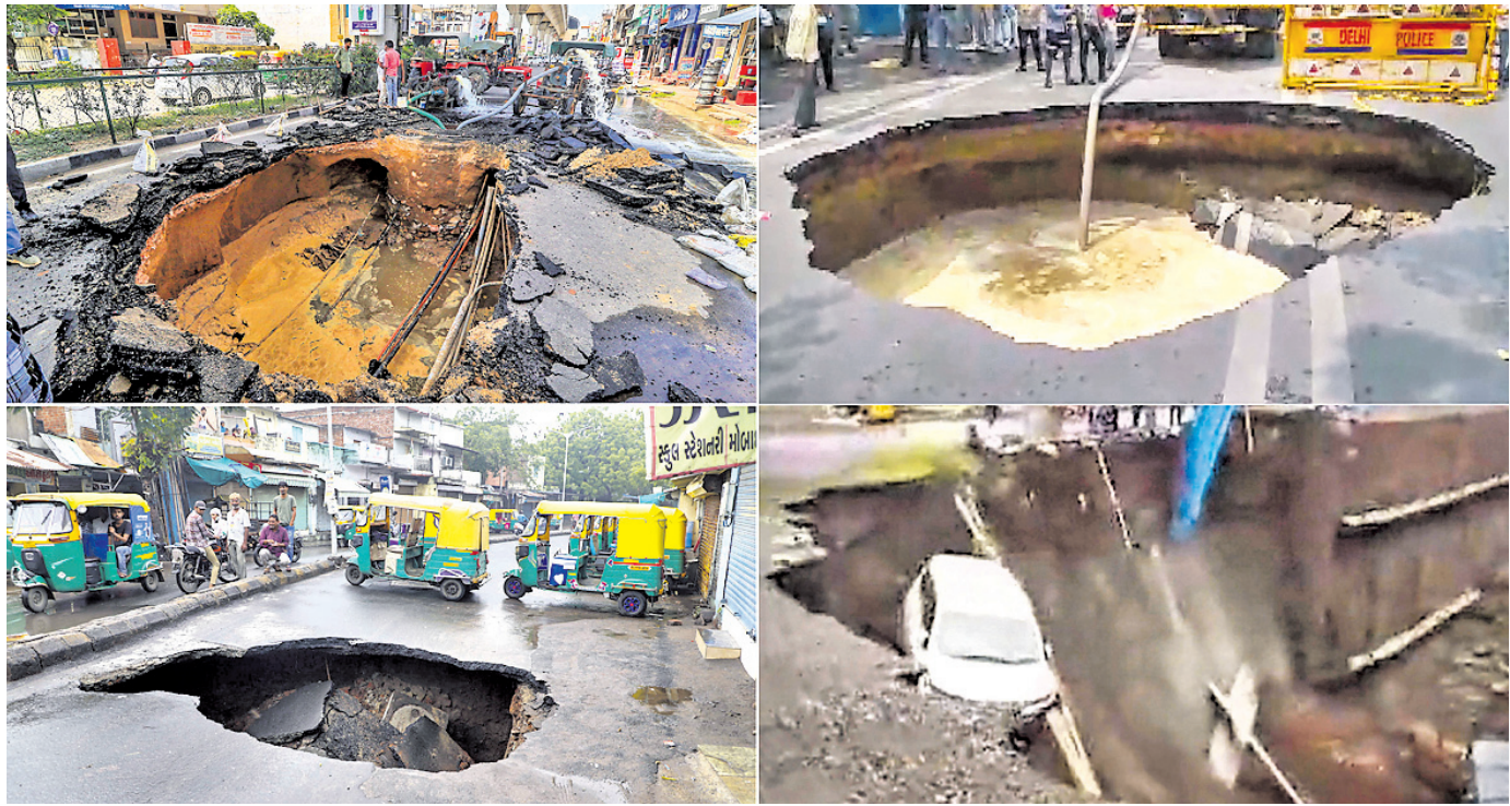
Combo picture shows craters formed on roads in Jaipur (top-L), New Delhi (top-R), Ahmedabad (bottom-L) and Mumbai, owing to rains
