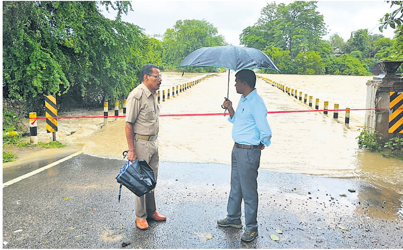
INUNDATED: The Poteru bridge over NH-326 connecting Kalimela with the Malkangiri district headquarters was closed for traffic after over 2-feet rainwater overflowed on the bridge following incessant rainfall in Malkangiri district, Wednesday
