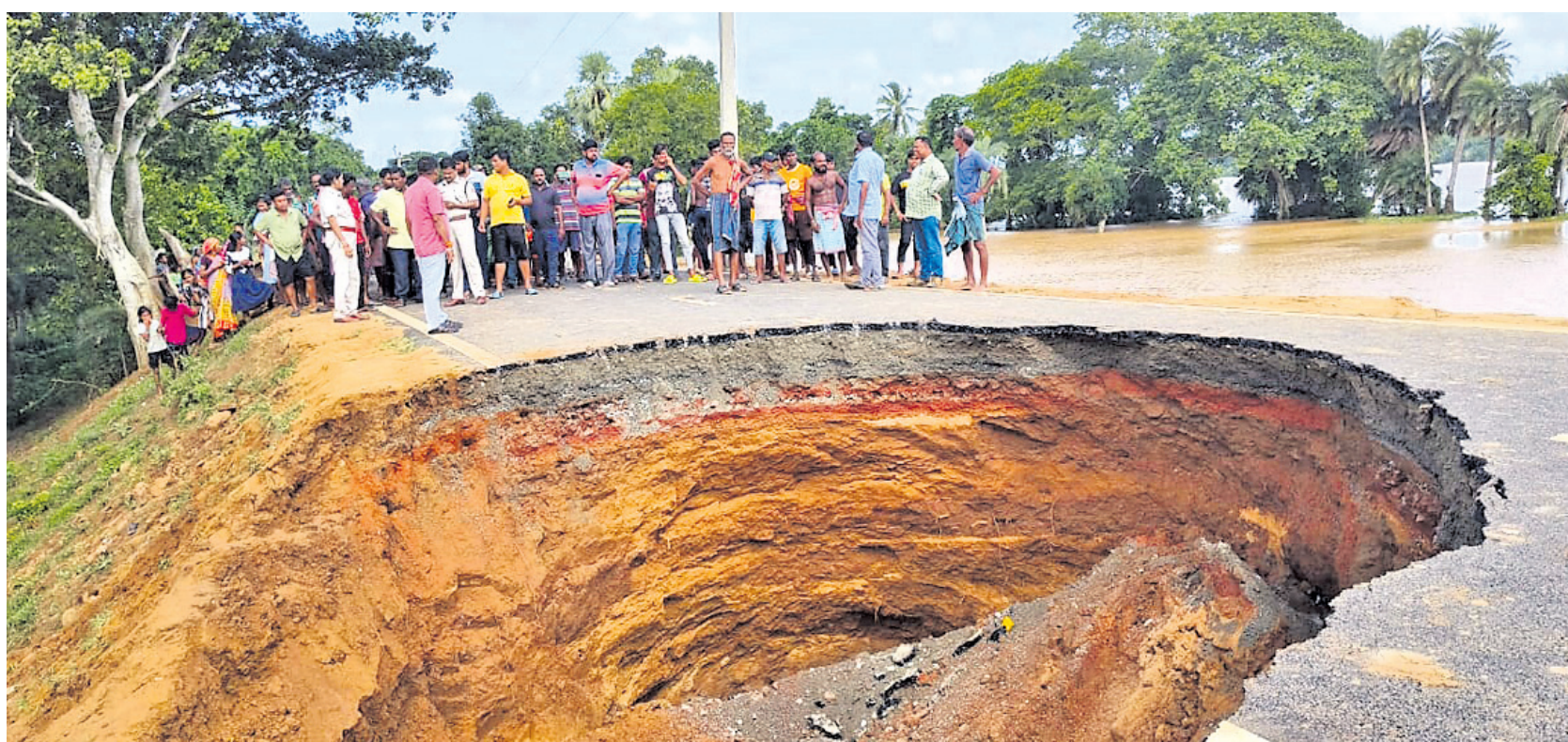
FLOOD FEAR: An embankment of Kharasrota river caved in after a sluice gate under it sank near Olei Chandanpur panchayat under Binjharpur block in Jajpur district, Thursday. This has sparked flood fear among the residents of riparian villages
