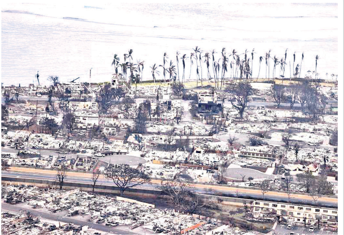
Fire damage is shown in the Wahikuli Terrace neighborhood in the fire ravaged town of Lahaina on the island of Maui in Hawaii
