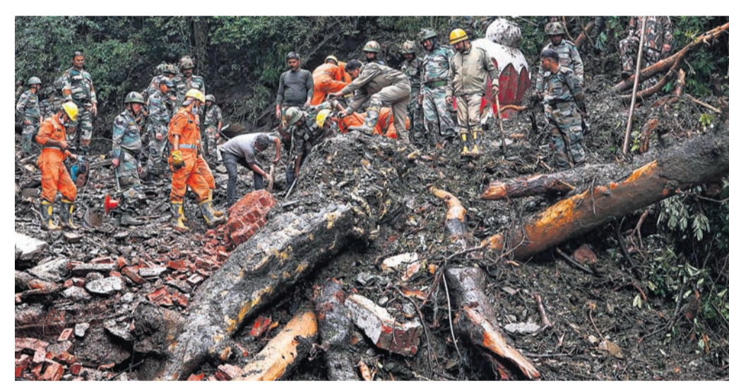
NATURE'S FURY: Army and NDRF personnel carry out rescue and relief work at the site of landslide after incessant rains in Shimla, Himachal Pradesh. The death toll rose to 74 as another body was pulled out of the rubble of a Shiva temple here and two more people were killed in Chamba district
