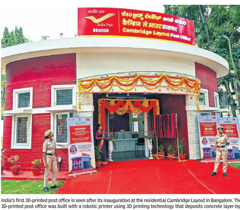
India's first 3D-printed post office is seen after its inauguration at the residential Cambridge Layout in Bangalore. The 3D-printed post office was built with a robotic printer using 3D printing technology that deposits concrete layer-by-layer in accordance with computerised 3D model drawing input
