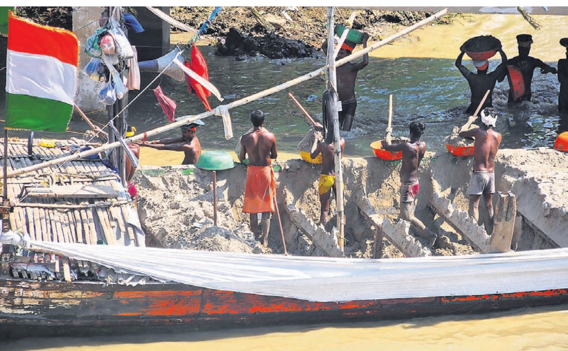
Workers unload sand from a boat despite state government's ban on sand mining, near Tekari ghat in Patna
