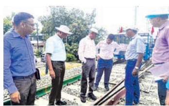
CRS inspects doubling work between Sambalpur City to Sambalpur (6.10 Km)
