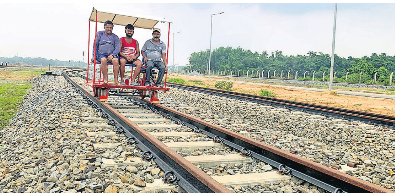
Trial run of motor trolley underway on India-Bangladesh railway line in Agartala
