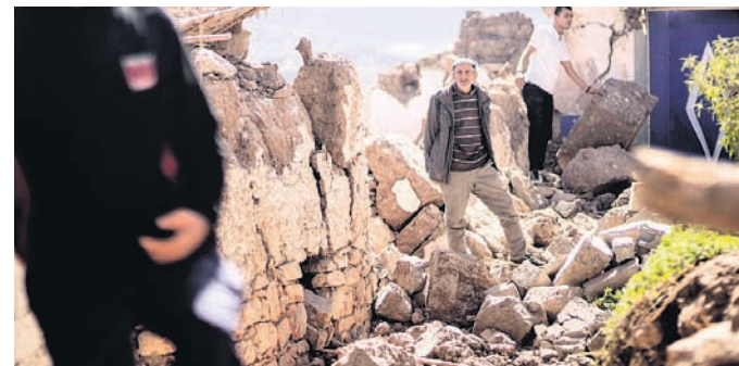
People inspect their damaged homes after an earthquake in Moulay Ibrahim village, near Marrakech, Morocco PTI PHOTO
