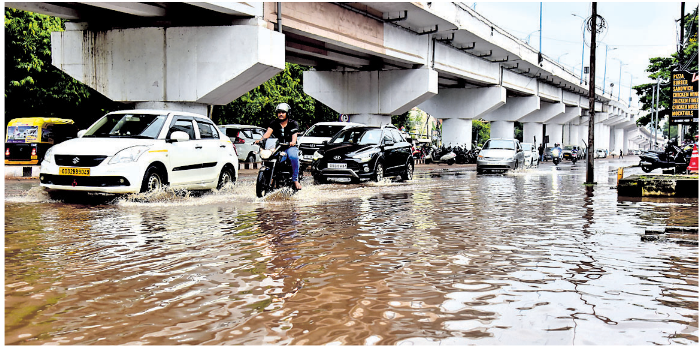
RAIN PAIN: Commuters negotiate a waterlogged Rasulgarh-Bomikhal Road after rain lashed Bhubaneswar, Monday
