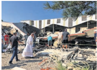
The Tamaulipas state police said about 100 people were in the church at the time of the collapse
