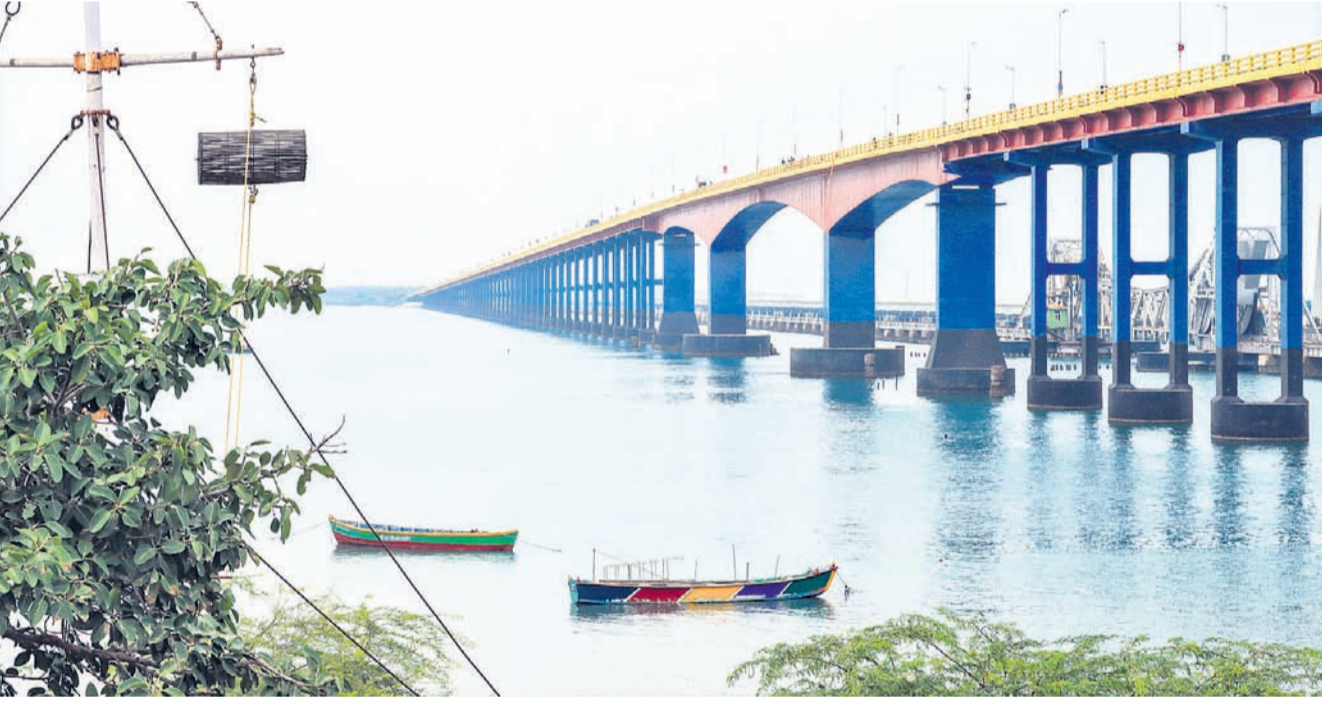
Pamban bridge near Rameshwaram, Sunday. IMD has forecast rains in coastal states after formation of a low-pressure area in Bay of Bengal
