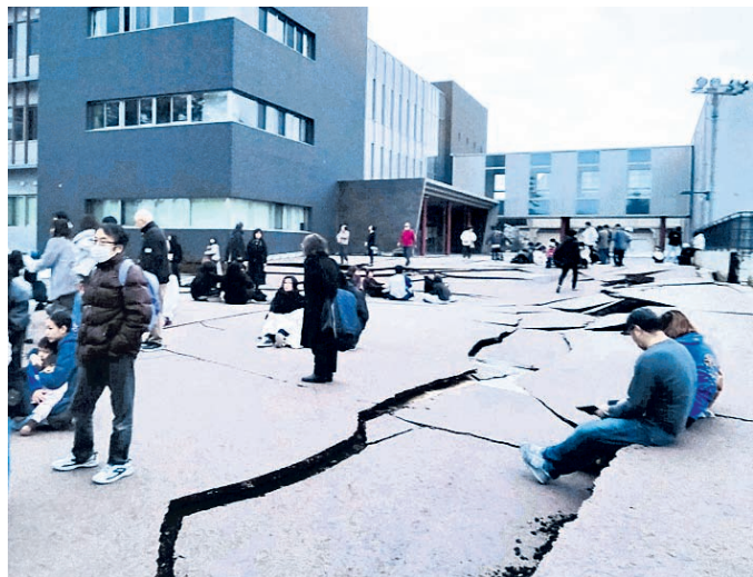
Cracks are seen on the ground in Wajima, Ishikawa prefecture, Japan
