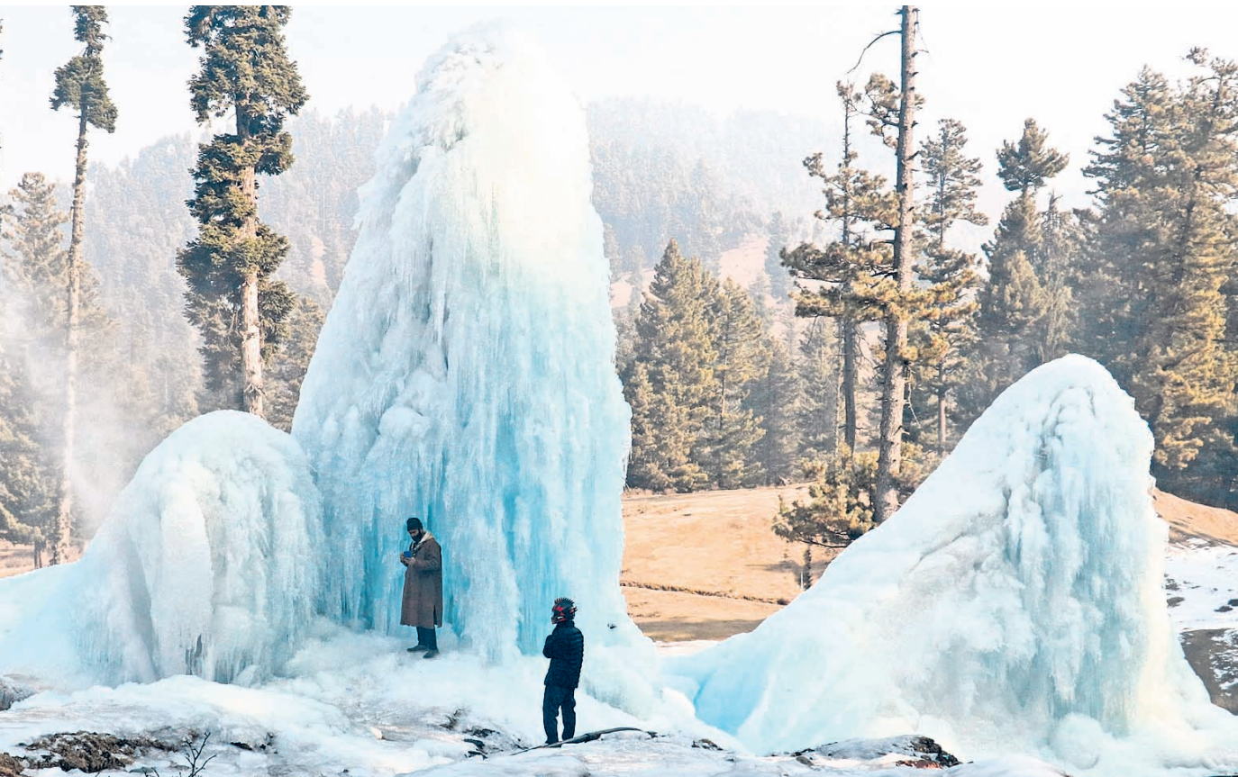
People stand near the long icicles formed after leak of a water pipeline at Tangmarg in north Kashmir
