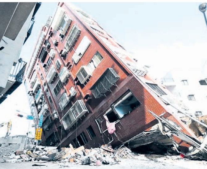
Debris surrounds a tilted building a day after a powerful earthquake struck in Hualien City, eastern Taiwan, April 4.
