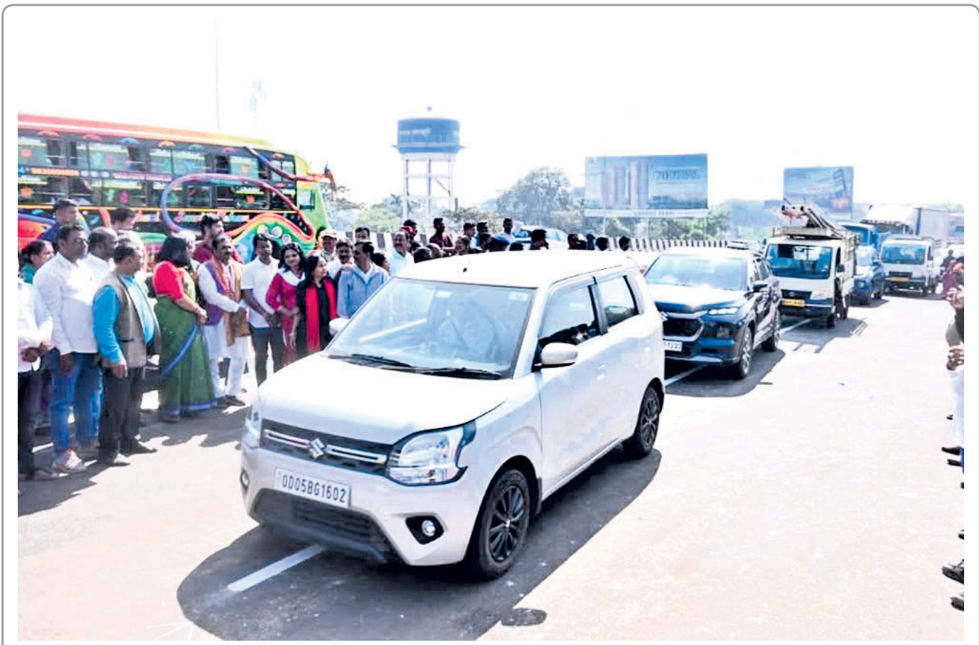
VITAL LINK: The much-awaited Hanspal flyover, constructed at a cost of ₹24.5 crore, was thrown open to public by Bhubaneswar MP Aparajita Sarangi Tuesday
