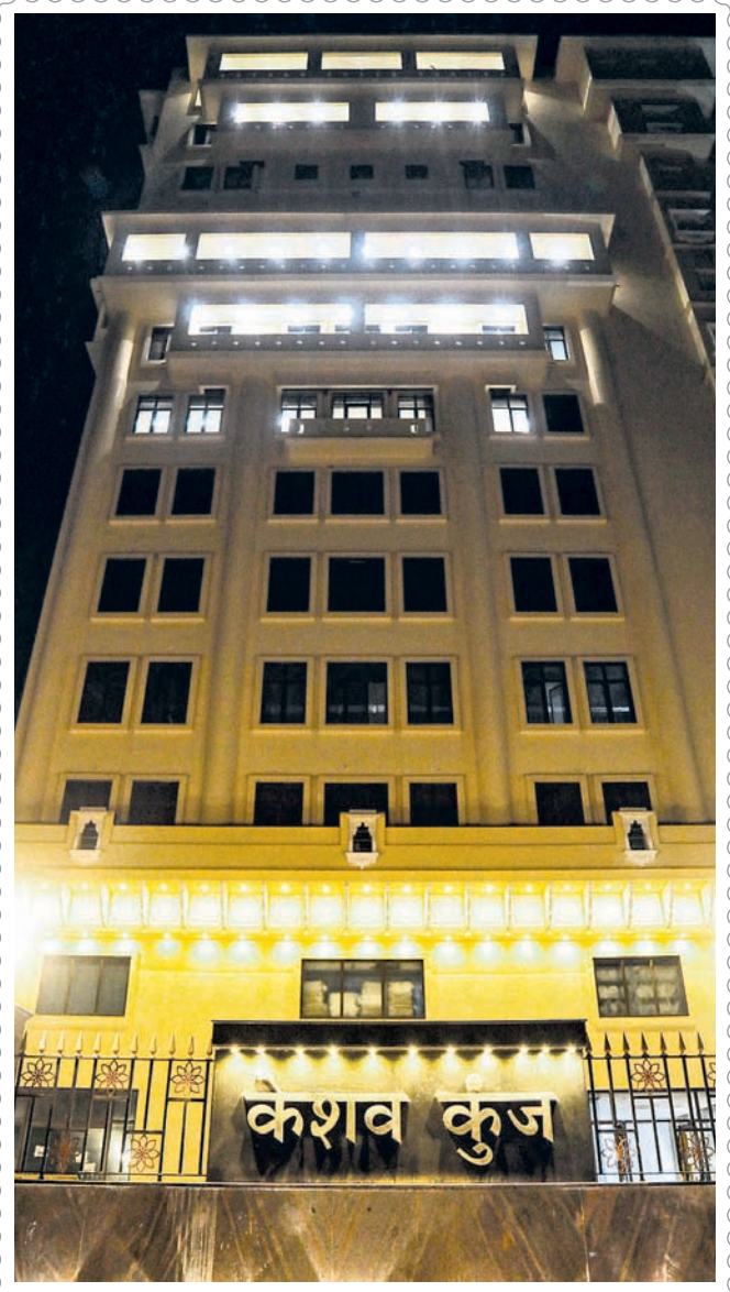
View of the rebuilt Rashtriya Swayamsevak Sangh (RSS) office, Keshav Kunj, at Jhandewalan, in New Delhi. RSS has moved back its office in the city to its old address following the near completion of the rebuilding project spread across over 3.75 acre premises, housing three 13-storey towers and around 300 rooms and offices in total
