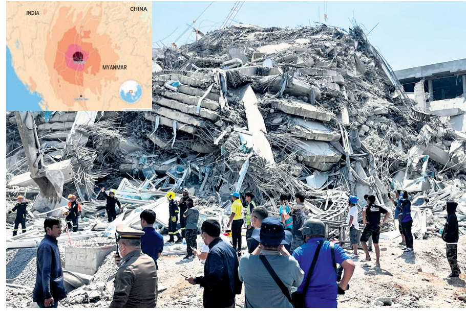
DEVASTATION: People stand near the site of a collapsed building in Bangkok, Thailand, Friday
