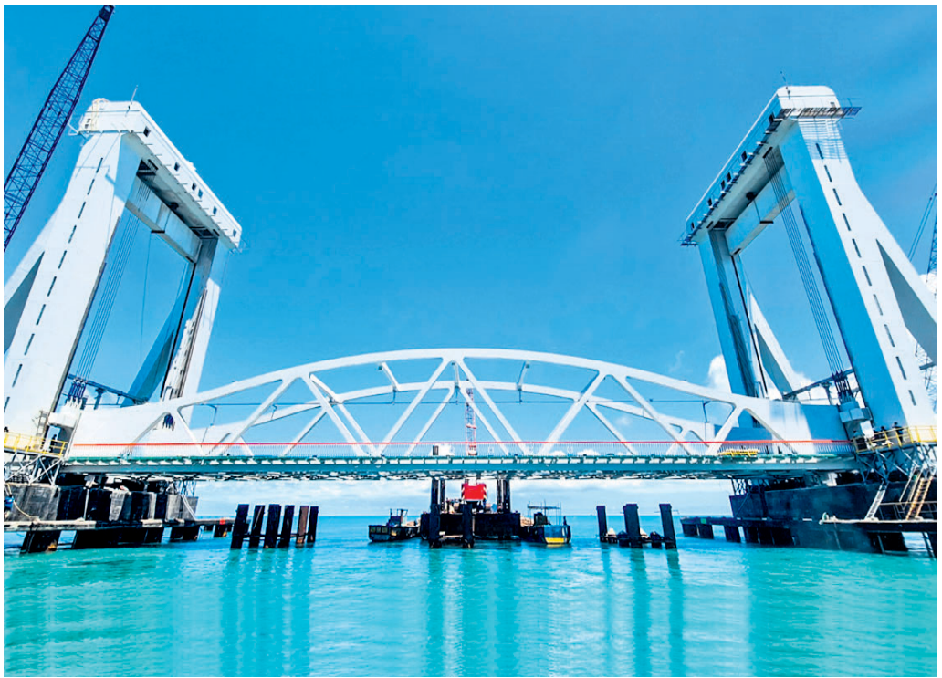
The new Pamban Bridge, connecting Rameswaram with mainland India, that will be inaugurated by Prime Minister Narendra Modi on Ram Navami (April 6), at Rameswaram in Ramanathapuram district of Tamil Nadu. It is considered to be India's First Vertical Lift Railway Sea Bridge PTI PHOTO
