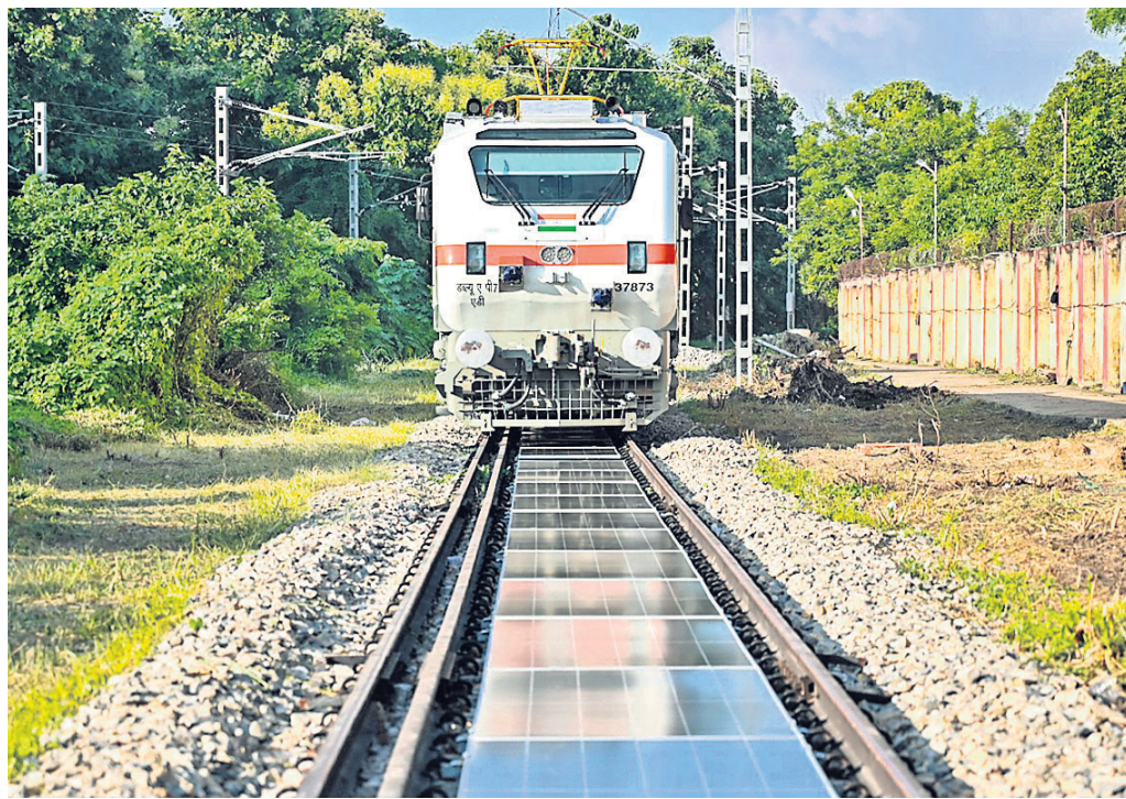
Banaras Locomotive Works, Varanasi commissioned India's first 70m removable solar panel system, 28 panels, 15KWp, between railway tracks PTI PHOTO
