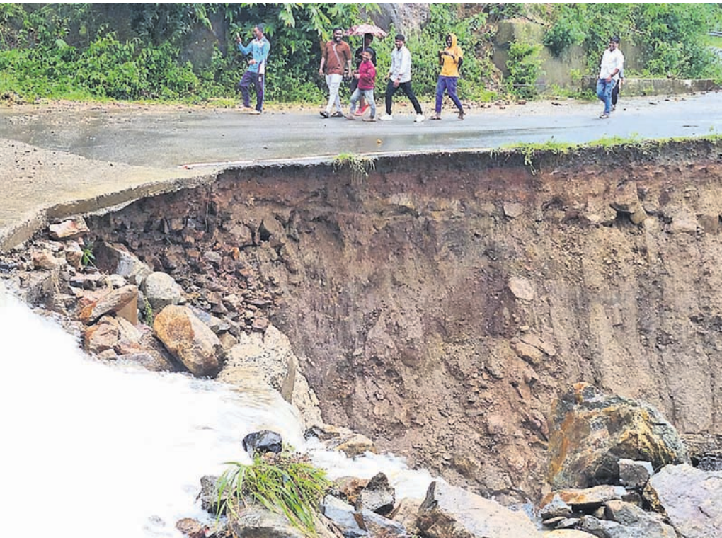
DEVASTATING IMPACT: A large crater was formed on the road near Mangadjhola village connecting Bonda Ghati in Khairput block of Malkangiri district after a landslide triggered by heavy rainfall washed away a major portion of the road Monday
