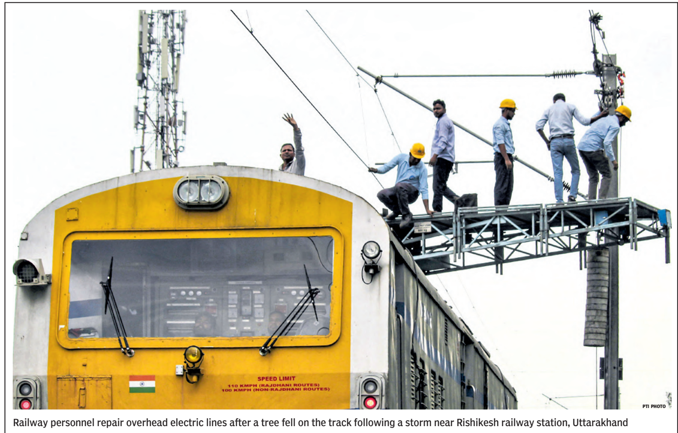
Railway personnel repair overhead electric lines after a tree fell on the track following a storm near Rishikesh railway station, Uttarakhand
