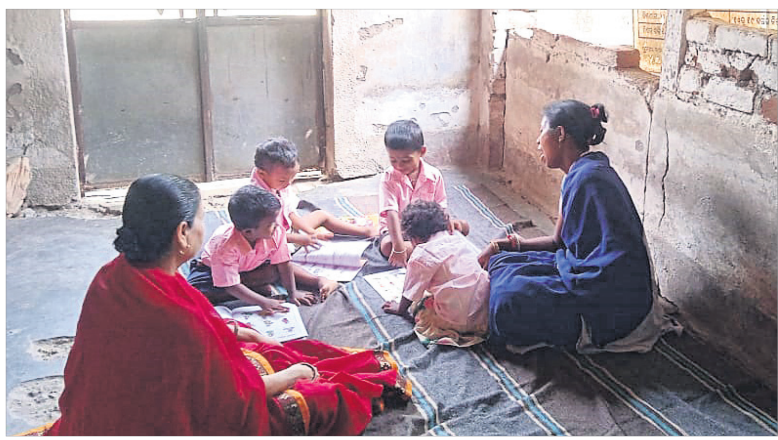
FUTURE IN PERIL: Children at Durgapur under Mayurbhanj's Kaptipada block forced to study under unsafe conditions in a dilapidated house sans an Anganwadi Centre
